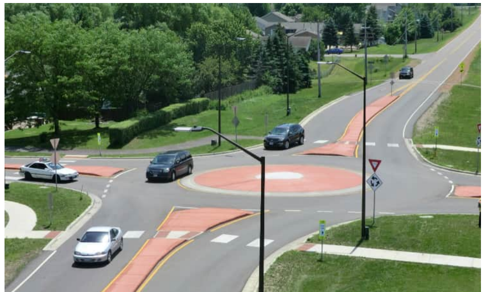
Example of a single-lane roundabout. Source: FHWA
