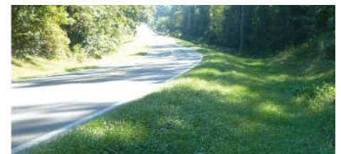
Clear zone provided on the outside of the curve. Source: FHWA.
