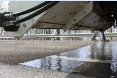
Automated application of HFST. Source: FHWA
