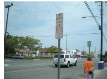
PICTURE 6: NO PARKING SIGNS WORN AND ON NON-BREAKAWAY POST, NORTH OF COLUMBINE ROAD
