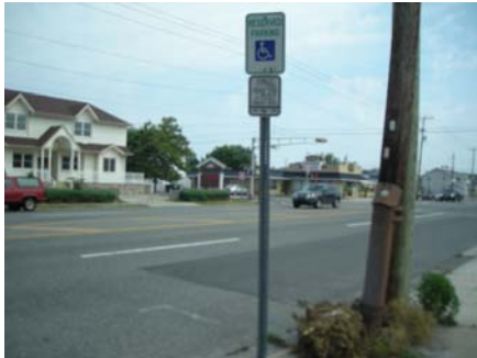
PICTURE 5: RESERVED PARKING SIGN POST NON-BREAKAWAY, SOUTH OF PALM ROAD
