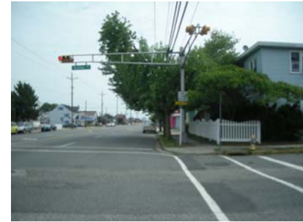
PICTURE 4: NON-BREAKAWAY SIGN AT LINCOLN AVENUE
